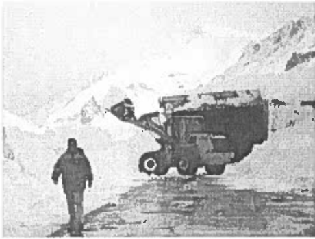
Even in avalanche areas snow has been easily removed due to anti-icing.
