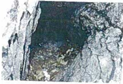
Close-up photo of cavity in central stem.
